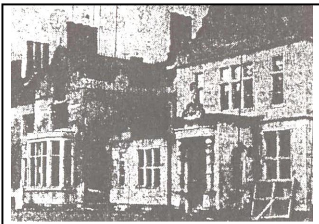
Demolition of the House
