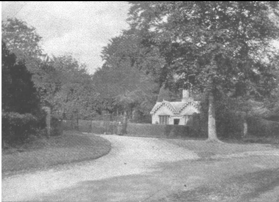
Lodge Cottage on Hardwick Lane, with the original gates
